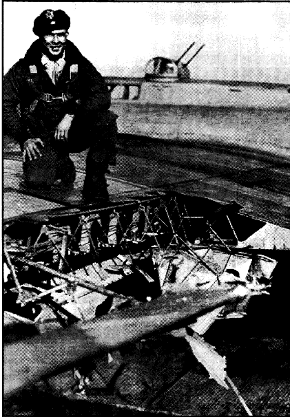
Inspecting cannon fire damage inflicted by German jet-powered fighter planes. Wing control surfaces were damaged but the fuel tanks remained intact as the pilot brought the B-17 back from the raid on Hamburg.
