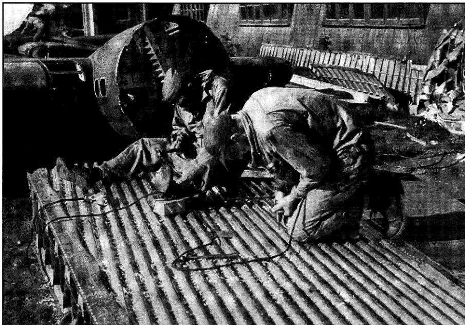
Stripping the metal skin from the wing of a crashed Fortress at a US Bomber station; to be used for minor repairs on mission damaged bombers.
