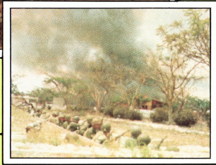
First Cracks: Quang Tri, 1972
